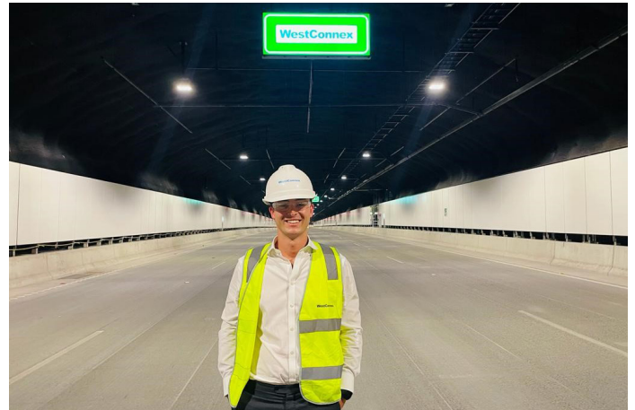
Figure 11: Sydney - Transurban's new M4-M8 Link Tunnel
