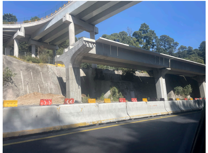
Figure 16: Slow progress on the Mexico City-Toluca train
