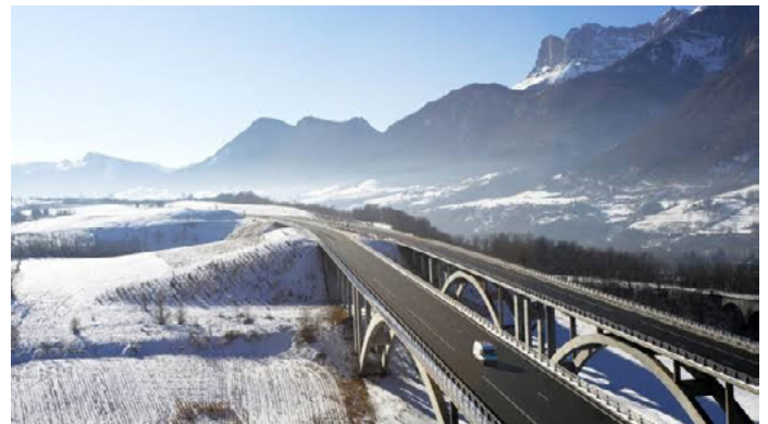
Figure 8: Eiffage & Atlas Arteria's APRR Network in France
